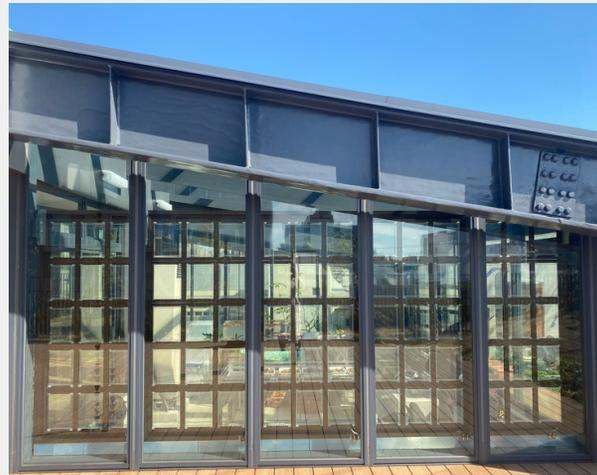
**Retrofit windows generating power from both outdoor & indoor light sources, heat shield as well**
